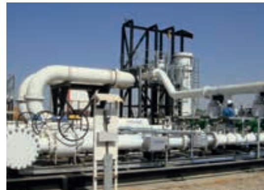
Skid mounted metering system with integrated ball prover
