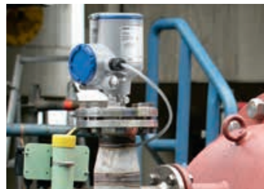
Butanol level measurement on bypass chamber
