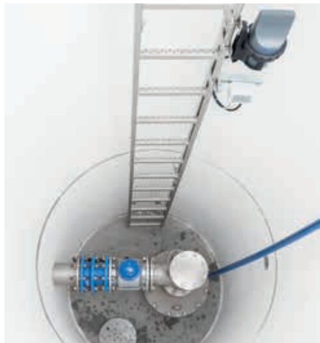
Battery-powered IP68 metering point with GSM/GPRS communication
