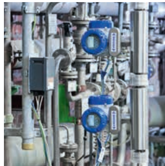
Straight tube coriolis meters in a safety application
