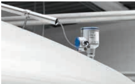
Level measurement on a milk tank
