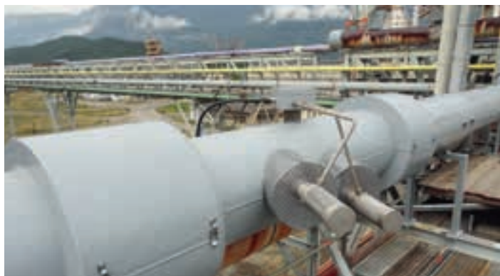
Ultrasonic flow measurement of superheated steam
