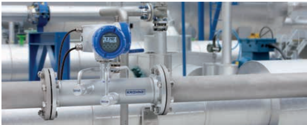
Process gas measurement with OPTISONIC 7300
