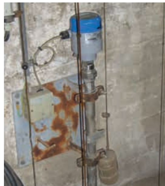
TDR level transmitter as overfill protection in water pit
