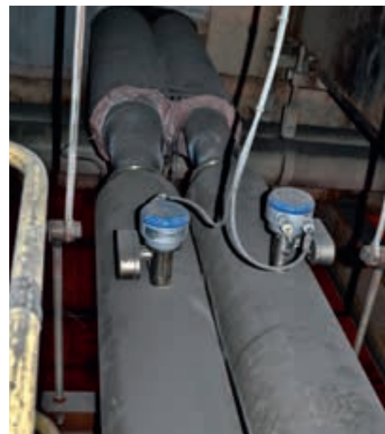
Mass flow measurement of heavy fuel oil
