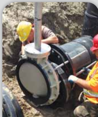
18" Polypropylene butterfly valves with stainless steel stem extensions for a landfill methane collection system
