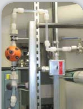
ChemFlare™ System (valves/fittings/tubing) and polypropylene back pressure/relief valves in a DI water system in the medical industry
