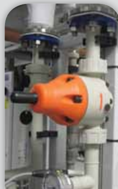
ChemFlare™ System (valves/fittings/tubing) and polypropylene back pressure/relief valves in a DI water system in the medical industry
