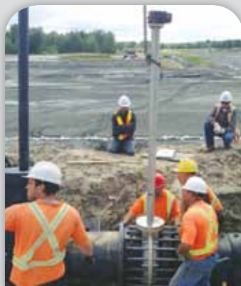
18" Polypropylene butterfly valves with stainless steel stem extensions for a landfill methane collection system
