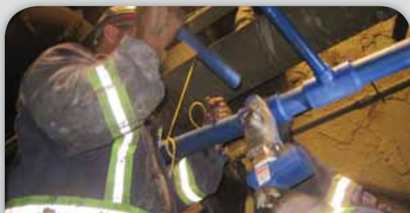
Installation of blue PE piping for compressed air in a copper mine operation
