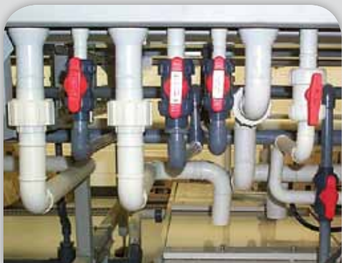
Polypropylene butt fusion piping system for high purity water in semiconductor industry
