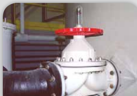
8" PVDF diaphragm valve for hot hydrochloric acid in a steel pickling line
